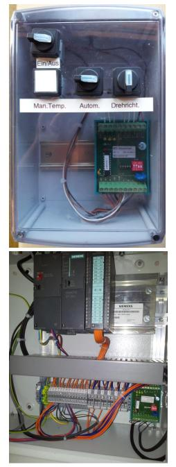
Installation of BPS-control unit in a plastic box as an autonomous unit (see 3.3 Application as autonomous unit).
